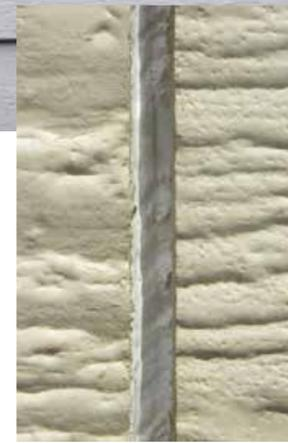
gaps at butt joints need caulk or clips which increasingly accentuate the gaps since they can fade at a different rate than the siding.
