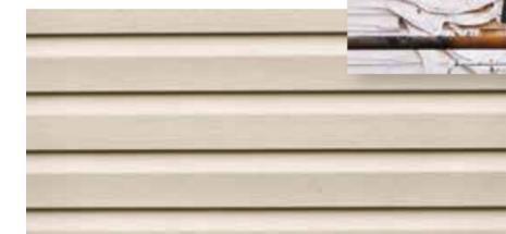
Vinyl siding is a plastic exterior that was introduced in the 1960s as an alternative to aluminum siding. While it certainly has plenty of merits in comparison to aluminum, vinyl siding comes with its own set of vulnerabilities: hail, the sun's UV rays, fire and heat can cause it to crack, buckle, warp—even melt.
