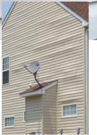
siding. Vinyl siding is installed in "panels" which create larger, more visible seams.
